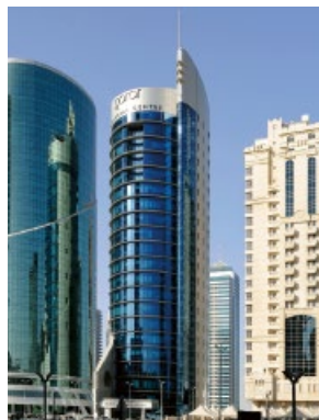
Doha, Qatar Financial Centre
